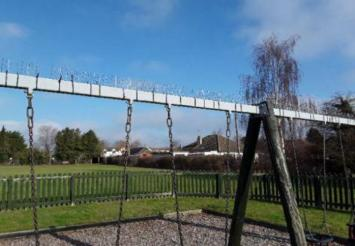
**Finding:** Steel bird deterrents have been used on the cross **Action:** Remove and replace with cable ties beam
