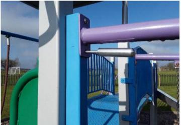
**Finding:** There is/are finger entrapment/s in the frame due Action: Replace the missing fixings to remove the to missing fixings and the item fails to meet the requirements entrapment of BS EN 1176 Part 1 4.2.7.6 Entrapment of fingers
